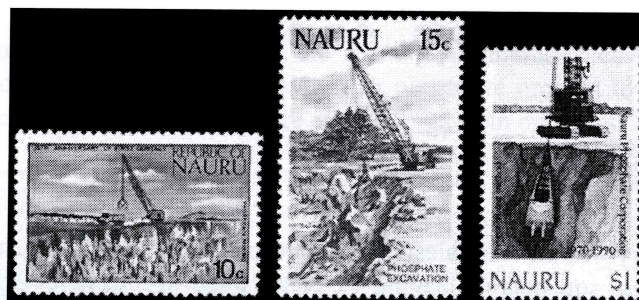
Excavation of the phosphate
